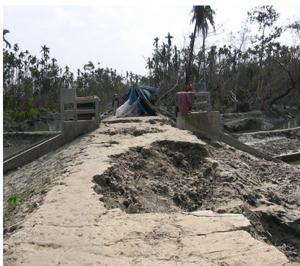
Fig. 4: Photo of damaged embankment by cyclone in Sidra in 2007
