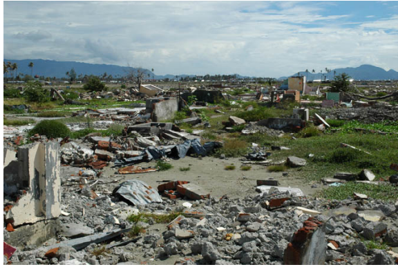
Fig.3 Destroyed buildings about 200 m inland from the coast
