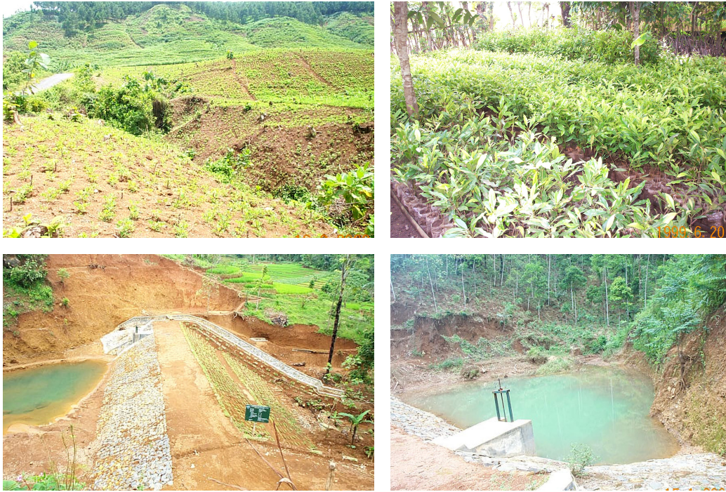
Figure 8. The activity of vegetative rehabilitation on critical land of upland area (top pictures) and mechanic method with check dam construction (below pictures).
