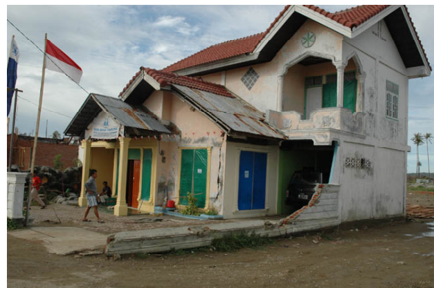
Fig.6 Destroyed building in the eastern part of the plain about 1.5 km inland from the coast
