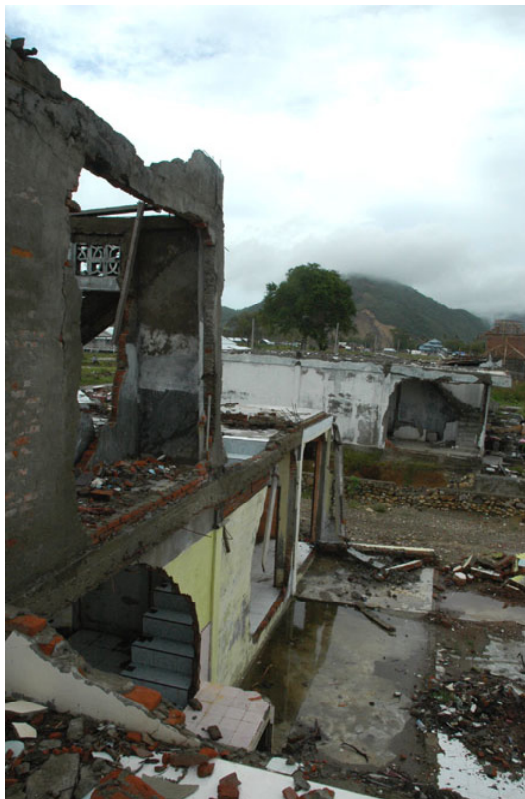
Fig.5 Destroyed buildings in the western part of the plain about 2 km inland from the coast
