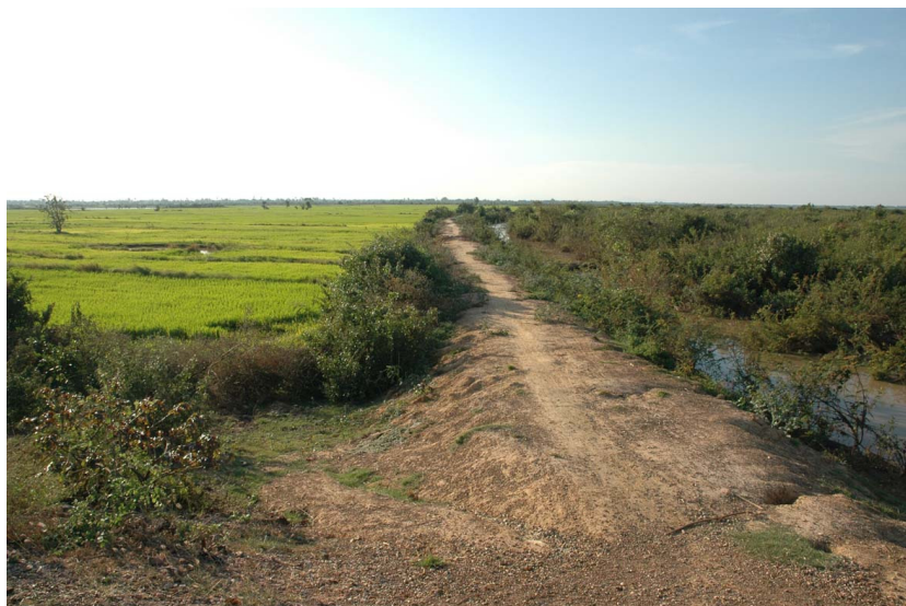
Fig.3b. A tomnup dike. Water is stored on the right side and used for paddy field on the left.
