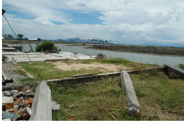
Fig. 8. Fallen columns indicating run-up tsunami direction
