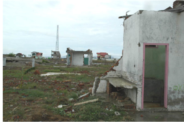
Fig.4 Destroyed buildings in the central part of the plain about 1.5 km inland from the coast
