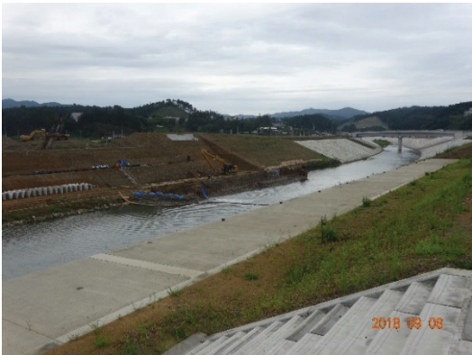
Figure 10. Embankment in Tohoku (Shizugawa in Minamisanriku town)
