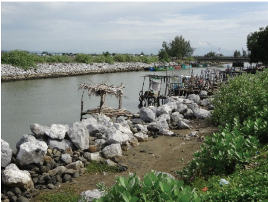
Figure 11. Embankment in Aceh (Alue naga in Banda Aceh)
